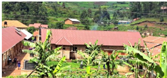
The Science Lab Nearly Completed
