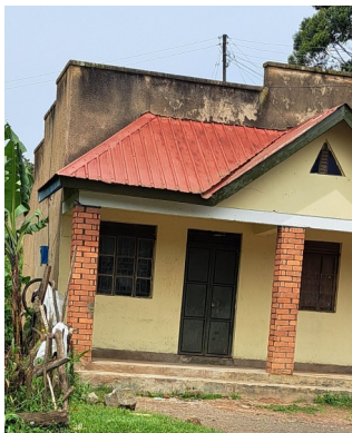
Refurbished Store Front
