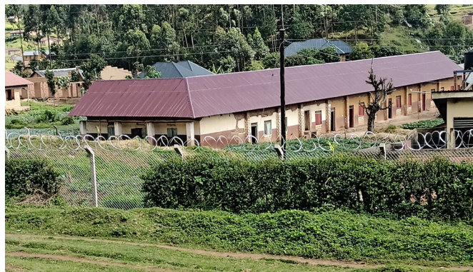
Section of the completed fence around the Muko High School Campus, made possible with funds provided by St. John's Episcopal Church Endowment Committee in Midland, Michigan
